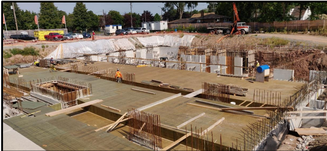
Forming the floor of parking level 1
