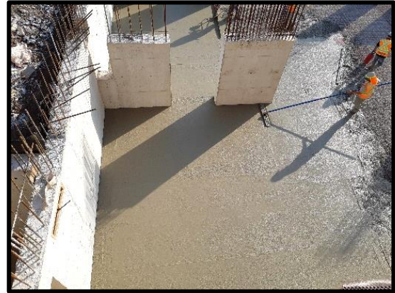
Pouring the floor of parking level 2
