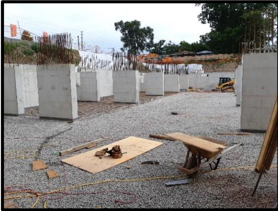
Preparing to pour the floor of parking level 2
