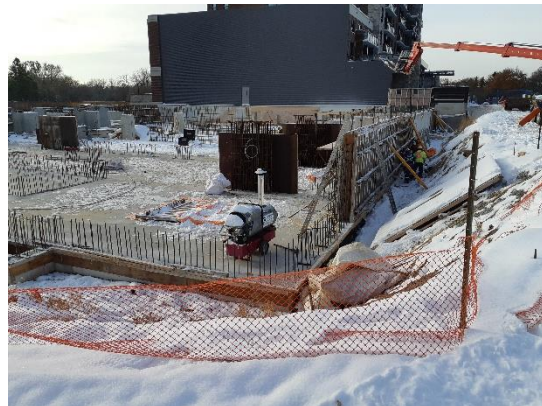
November 2019 – P1 and P2 Floor complete, P1 Walls started
